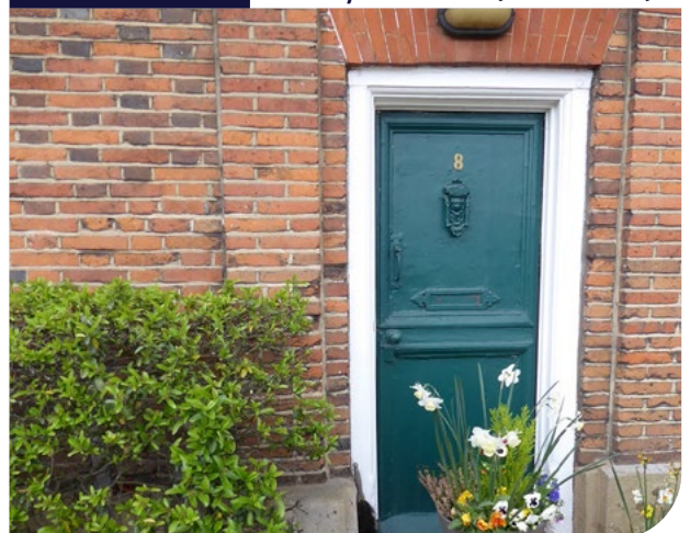
Detail of entrance to Winnocks Charity almshouse, Colchester, UK
