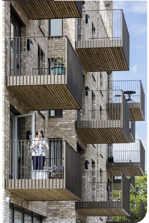
External balcony overlooking courtyard
